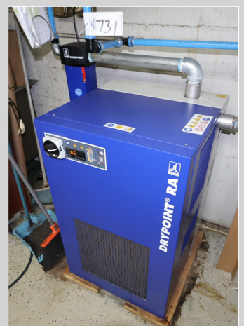
BEKO DRYPOINT RAX25N-E08 REFRIGERATION AIR DRYER
