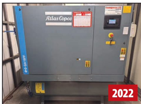
ATLAS COPCO GA15FF 20 HP AIR COMPRESSOR
