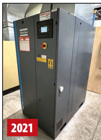
ATLAS COPCO GA37 50 HP AIR COMPRESSOR
