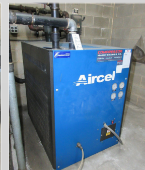
AIRCEL VF-500 REFRIGERATED COMPRESSED AIR DRYER
