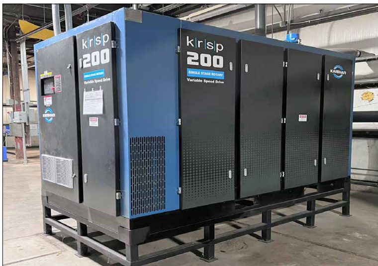
Kaishan KRSP-200 200-HP Rotary Screw Air Compressor
