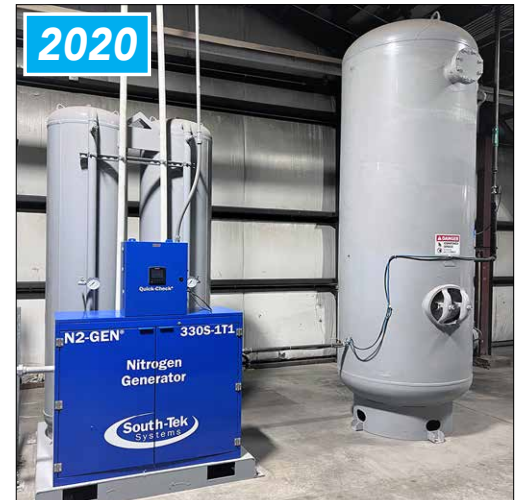
Southtek N2-GEN Nitrogen Generator System
