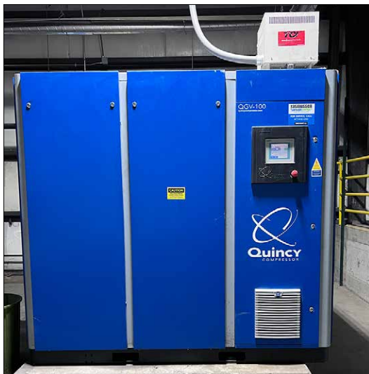
Quincy QGV-100 100-HP Rotary Screw Air Compressor
