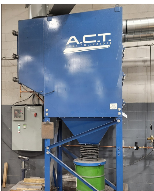
ACT (8) FILTER DUST COLLECTOR VIEW LOT #6A
