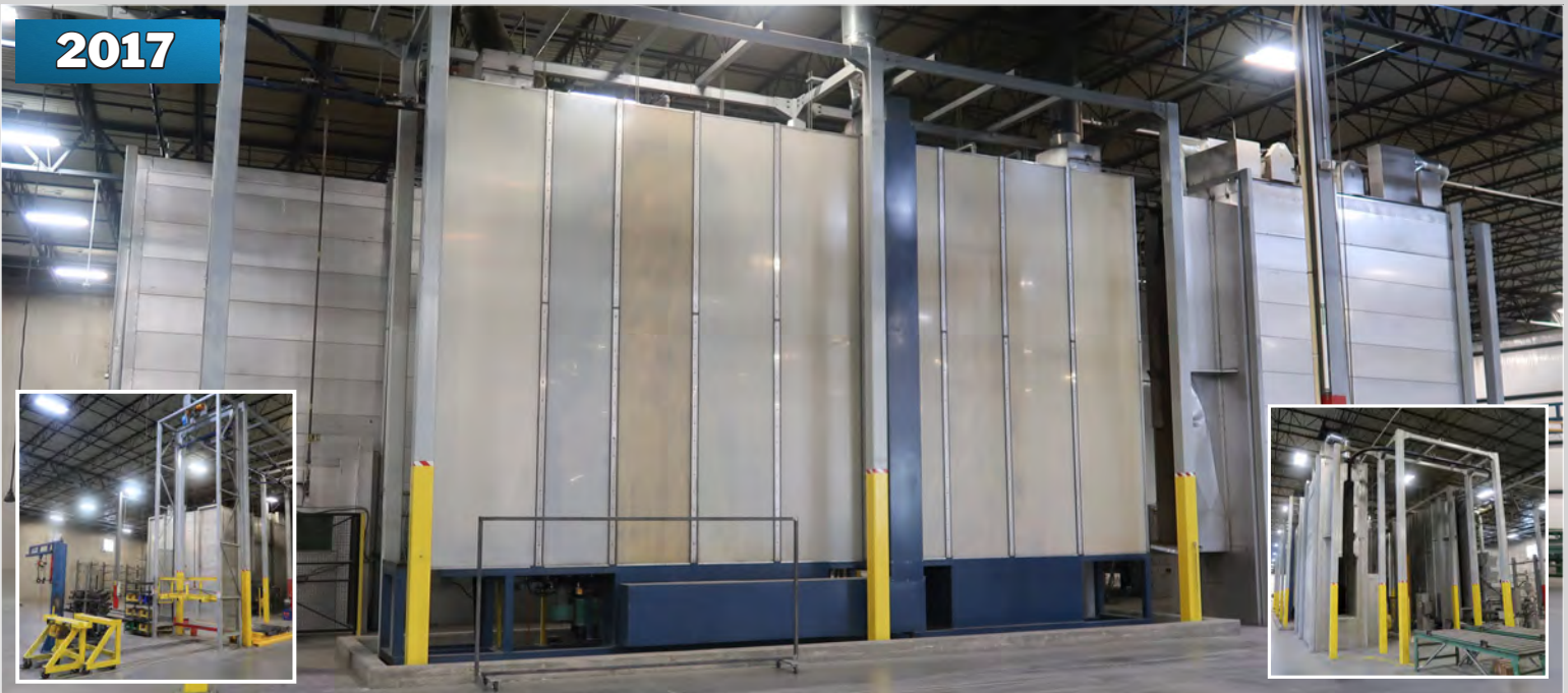
ROHNER DESIGN POWDER COAT PAINT LINE
