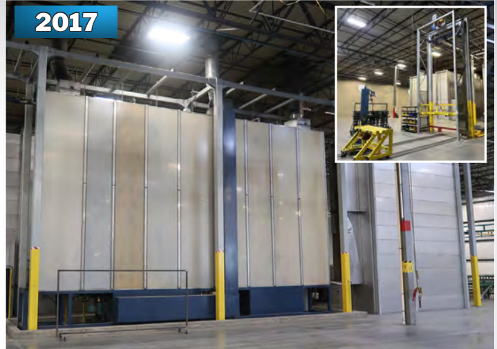
ROHNER DESIGN POWDER COAT PAINT LINE
