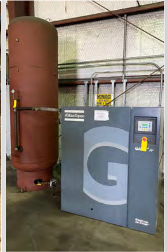
ATLAS COPCO AIR COMPRESSOR
