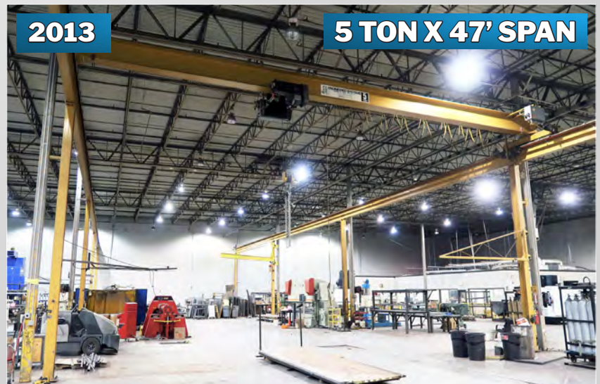
ENGINEERED SYSTEMS OVERHEAD BRIDGE CRANE
