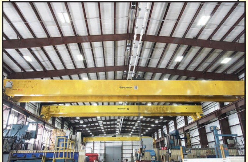
PROSERV 30 T. X 100' SPAN OVERHEAD BRIDGE CRANE
