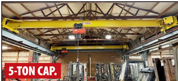
5-TON CAP. CRANE AMERICA 5-TON BRIDGE CRANES
