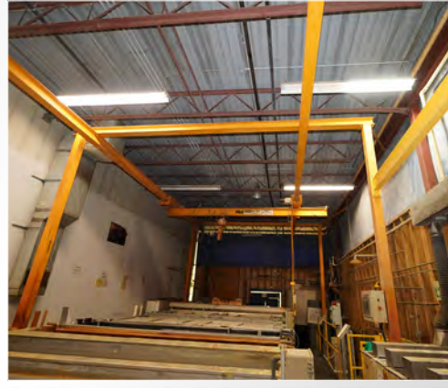
3-TON P & H MODEL 3 TRAVELLING BRIDGE CRANE
