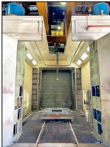
BINKS 10' X 28' X 16' WASH AND PAINT BOOTH
