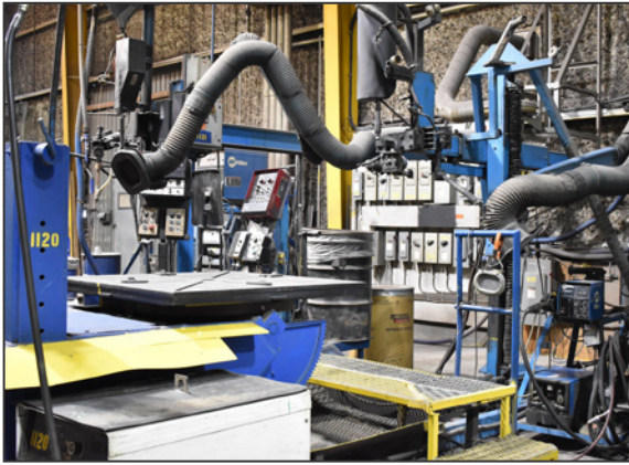
Partial view of subarc welding system with welding positioners
