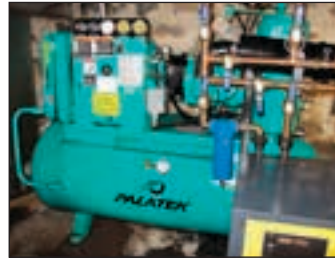
PALATEK 15 HP ROTARY SCREW AIR COMPRESSOR MODEL 15D
