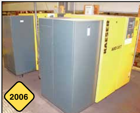
30 HP Kaeser ASD30T Compressor
