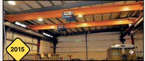
10-Ton Altoona/DeMag Radio Controlled Overhead Bridge Cranes
