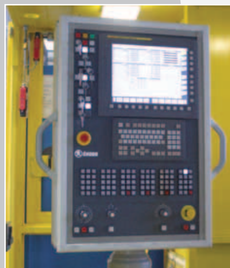
Main control panel GE FANUC 31i
