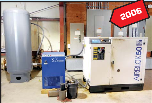
< AIRBLOK 50 HP ROTARY SCREW AIR COMPRESSOR, QUINCY DRYER AND RECEIVER
