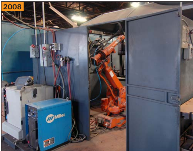
ABB 6 axis automated welding cell
