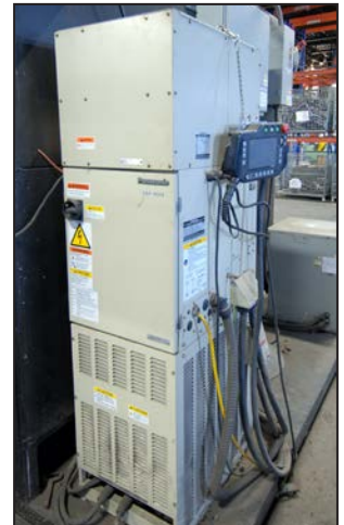
View of robot controls & pendant
