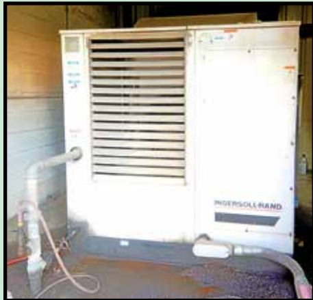
< INGERSOLL RAND 100 HP ROTARY SCREW AIR COMPRESSOR
