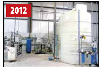
SECONDARY RO WASTE WATER TREATMENT SYSTEM
