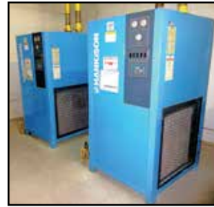
(2) HANKISON AIR DRYERS
