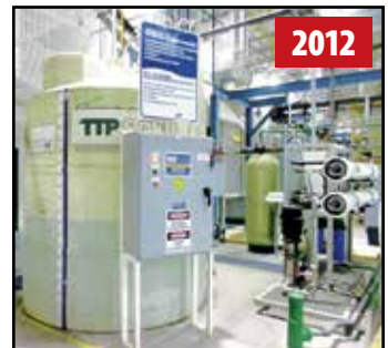
RO WASTE WATER TREATMENT SYSTEM
