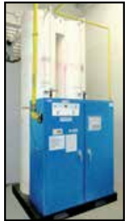
ON-SITE GAS SYSTEM NITROGEN GENERATOR
