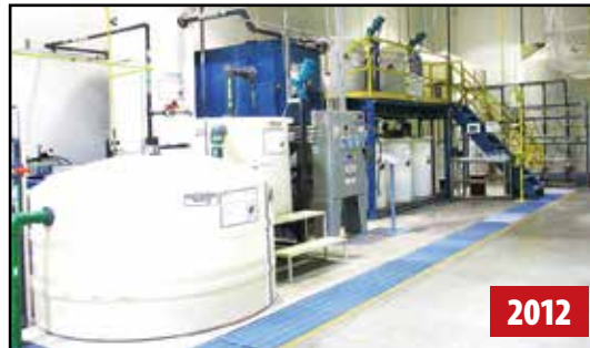
WASTE WATER TREATMENT SYSTEM
