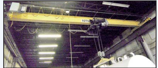
10-Ton Capacity Overhead Bridge Crane
