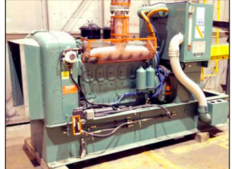
DETROIT DIESEL ALLISON DDACE-100 diesel generator
